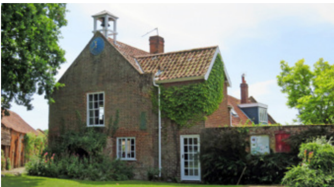
Converted school room located in the Village Green.
