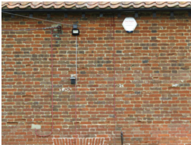
Accumulation of cables, light and security alarm
