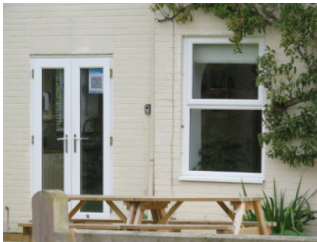
Inappropriate uPVC door and window
