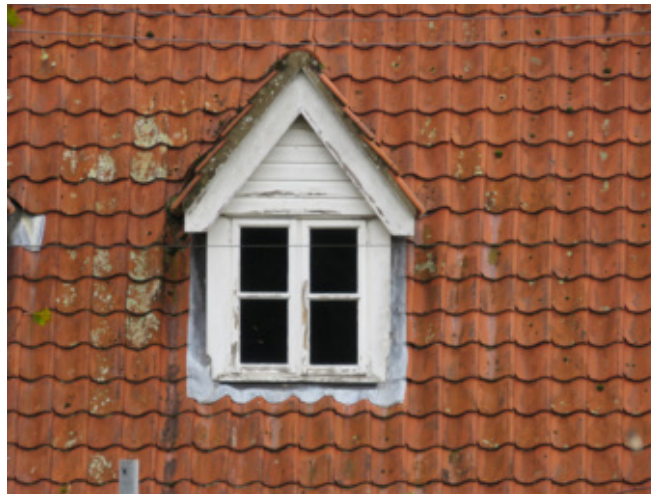
Window joinery that requires repainting
