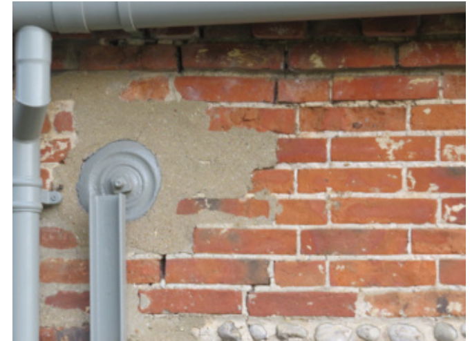
Cementitious repointing to brickwork
