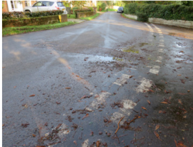
Patched road surface
