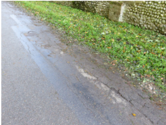
Poor road surface on The Street
