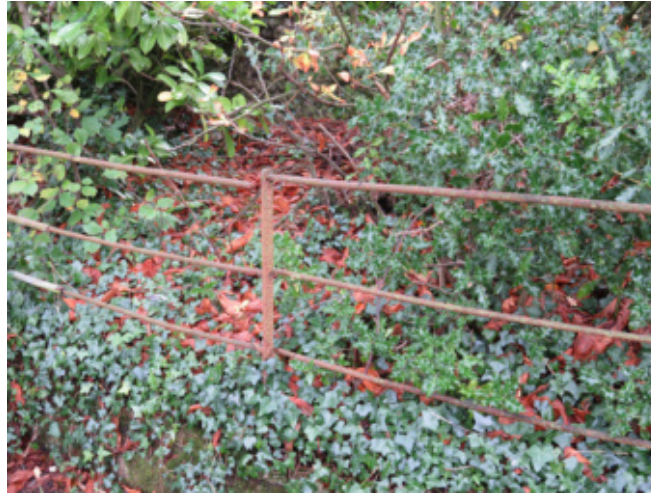
Metal railing to the churchyard
