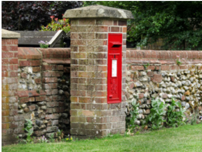
Wall post box on the east side of The Street near to the phone box
