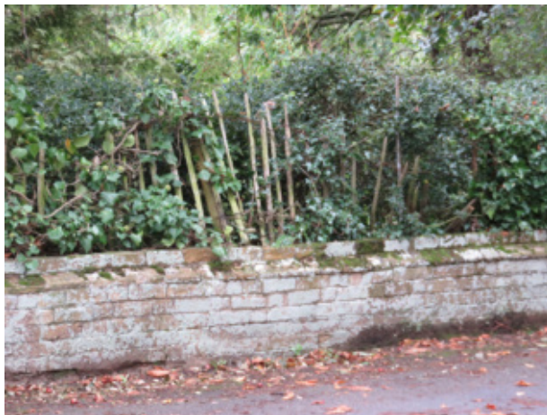
Post and wire replacement fence
