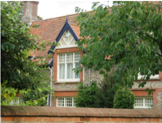
Gabled window on The Grange
