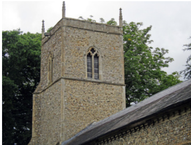
Detailed view of the church tower
