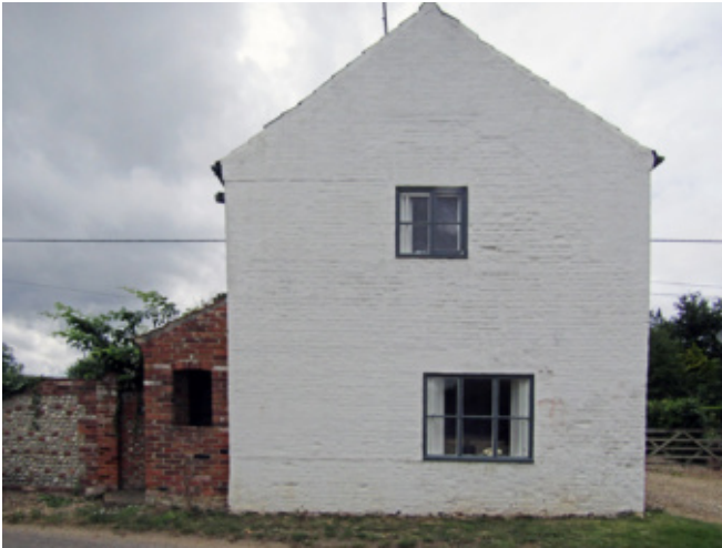
Cottage located north of The Street
