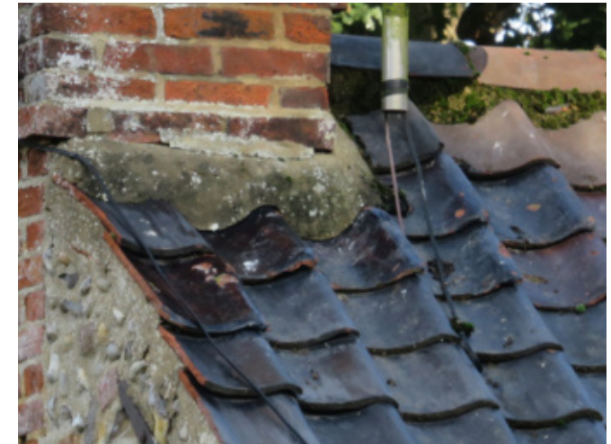
Inappropriate cementitious repairs to chimney and roof
