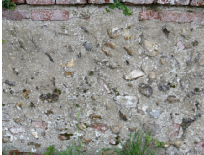
Excessive repointing to flint wall
