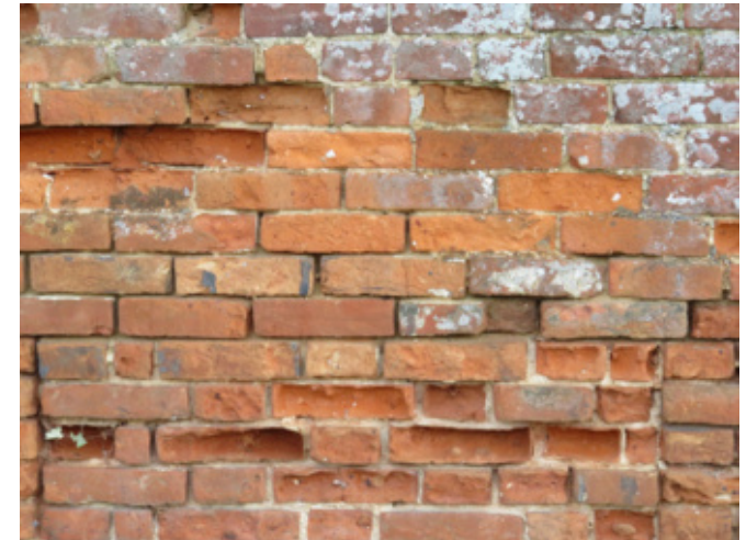
Eroding brickwork
