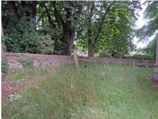
Cobble flint and red brick wall enclosing the churchyard with mature trees and shrubs beyond
