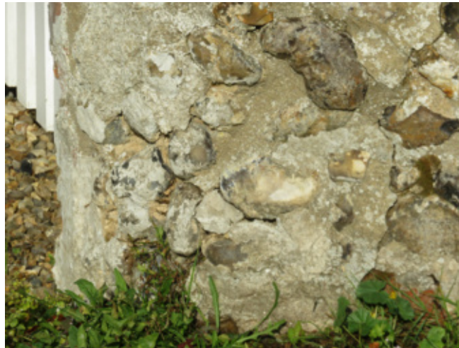
Cementitious pointing to a flint wall
