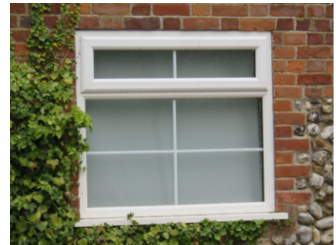
Inappropriate uPVC window
