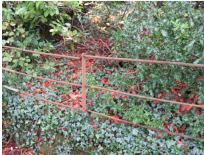
Broken and corroding railings
